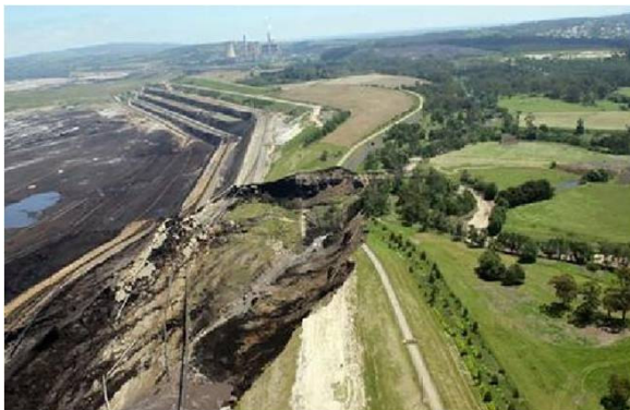
Mining alongside the Latrobe River ended in disaster. The Yallourn Mine Batter Failure Inquiry Report, June 2008, identified slack and lapsed safety standards and found that mine consultants had lacked the skill to give competent advice for more than a decade.
